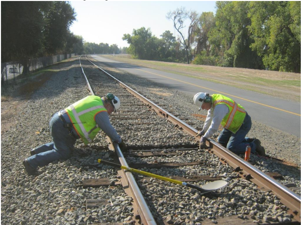
Frank and Steve install a gauge rod
