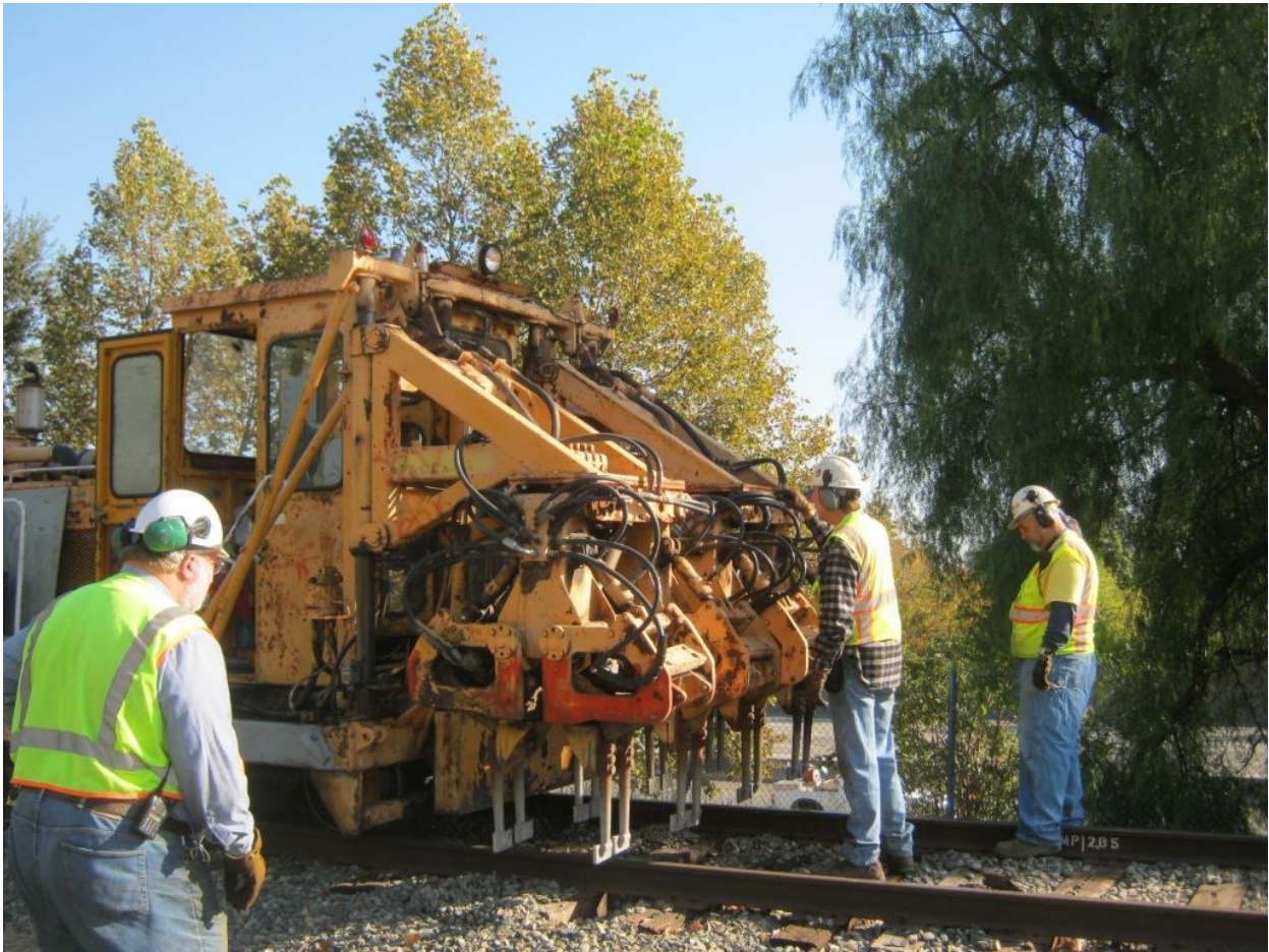
Straightening skewed ties was the first order of business
